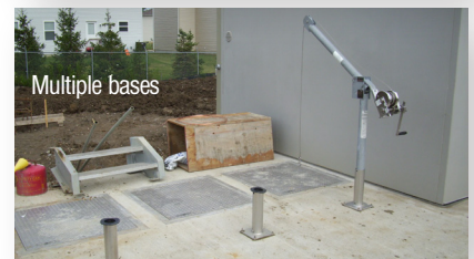
Pump/mixer lifting
